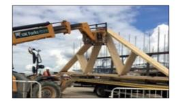
10. Metalwork bags must be removed from the trailer in conjunction with the driver's specific manual handling training. All other items to be removed by the forklift truck should be completed by following site procedures.
