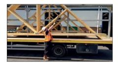
7. When instructed that the area is clear the forklift truck operator shall remove the trusses from the lorry.
