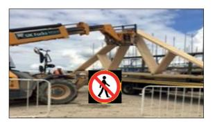
6. The driver can assist the responsible person to cut the individual 8mm blue rope attaching the bundle to the lorry. This should be completed from the ground using the telescopic tree cutters provided. The driver must be in a safe position when carrying out this function.
