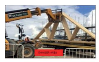
9. The forklift truck operator must lift the trusses from the trailer and then move the trusses to a safe off-load area. If the driver has to mount vehicle, he must do so under the authority and supervision of the site manager/contractor using agreed method of working at height safety equipment.
