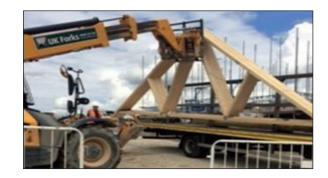
8. **NEVER** stand in the area around the lorry, or where the forklift truck will move into, or allow any others to enter the danger area.
