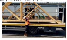
3. The FLT Operator must position the forks in the most appropriate area to lift the trusses safely. The forklift truck will take the weight of the trusses on the forks.
